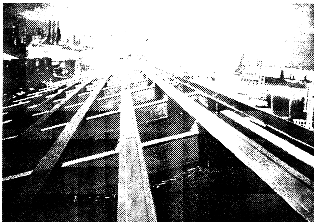
Figure 7. Caustic chlorine facility with spans up to 5.8 m and loads up to 1.9 KPa. Diamond Shemarock, Houston, TX. (Courtesy of Composite Technology, Forth Worth, TX.)
