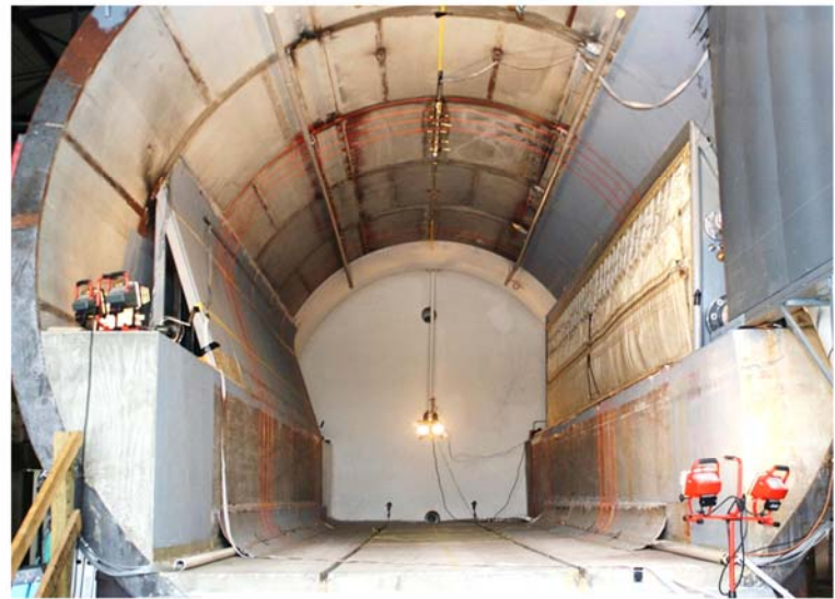
Tunnel Section Before Deployment
