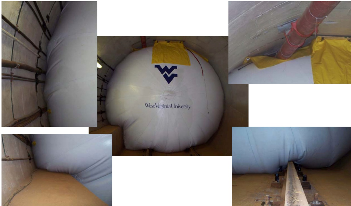
Figure 9: Seal provided by the plug to the different elements existing in the tunnel
