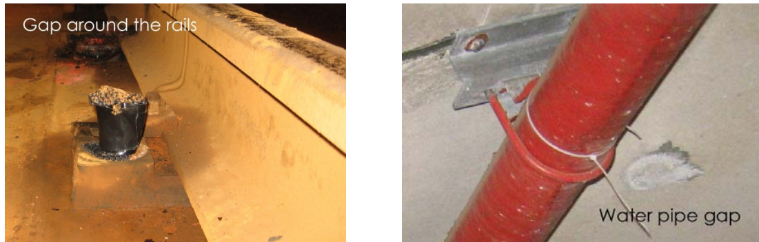
Figure 10: Existing gaps around rails and pipe
